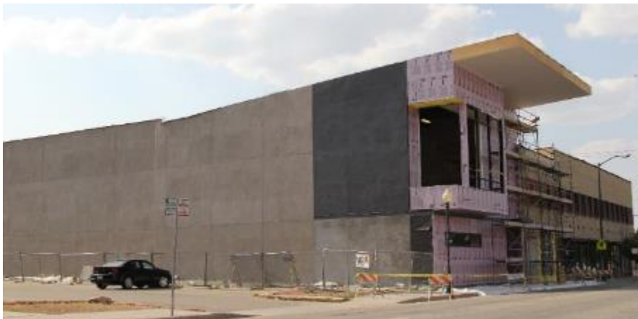
Construction photo from June 2014
